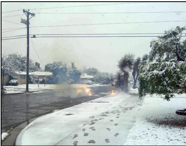
Downed power lines create hazardous conditions.
