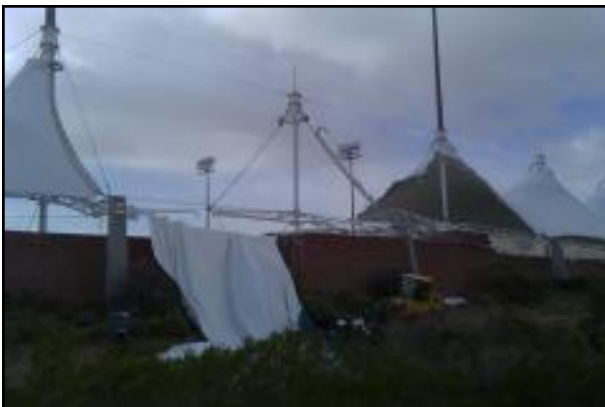
High winds damage Cohen Stadium Photo courtesy of KFOXTV.com 2009
