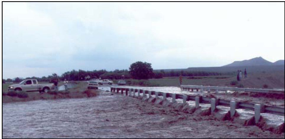
Placitas Arroyo overtops Channel Road, Hatch, NM, 2002; Photo by Hatch resident
